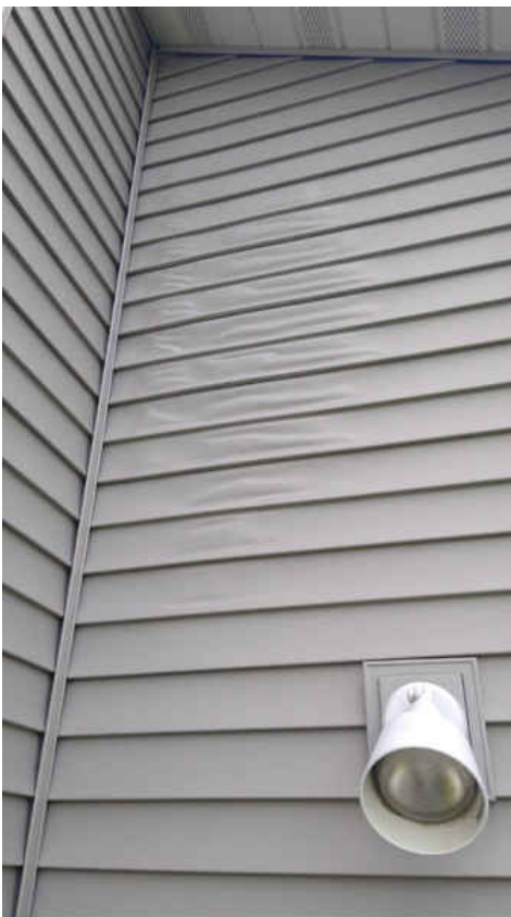
Damaged siding by Garage Walk-in Door
